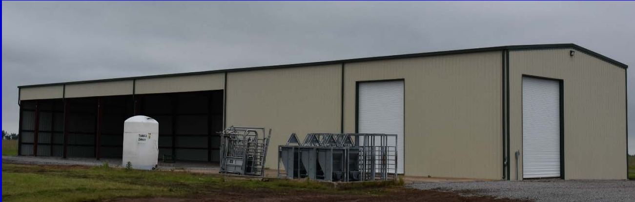
New Feed Mixing Facility
