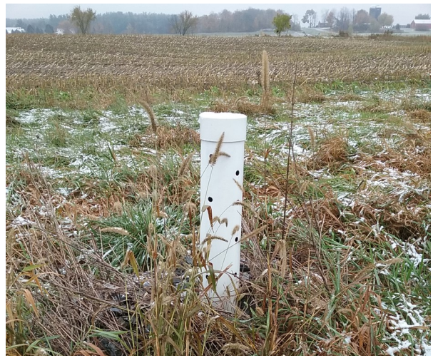
Image 1. Surface inlet with 25-foot buffer. (Photo courtesy of VAAFM)
